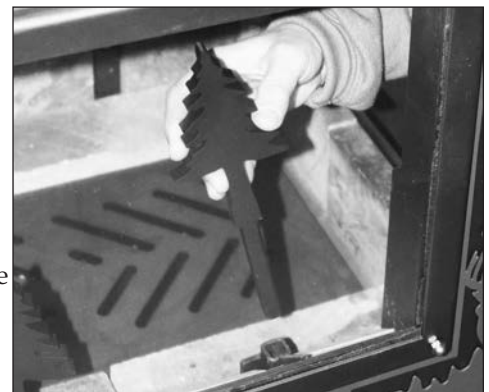
Insert the andirons back into the stove after cleaning the glass. The andirons help keep wood away from the glass and the air wash system unobstructed.
