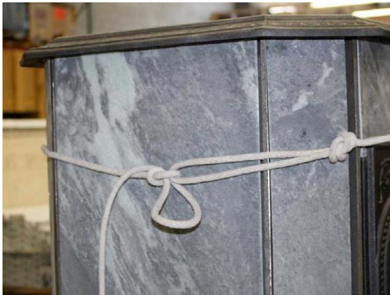
9. Remove the exterior stone panel. The furnace cement will make this removal difficult. If you rock the panel left and right as you lift it will help loosen the cement.
