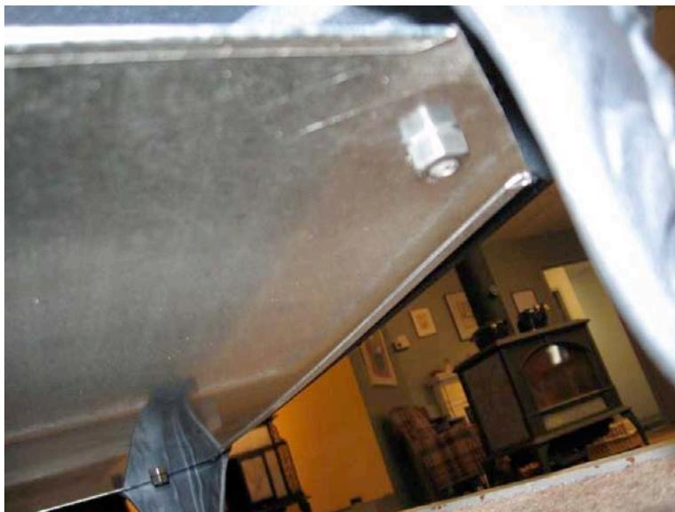
3. Raise the legs of the stove 2" off the floor. You may suspend the stove by placing something sturdy under the center of the stove or by placing wood under the two edges of the stove along the base.
