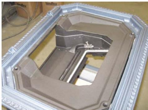
24. Install the four flat head screws into the air duct cover as follows: 2" in the right front, 4" in the left rear, and 5" into the last two, tighten.
