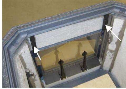
15. Install the eyebolts and tighten with a 9/16" socket.
