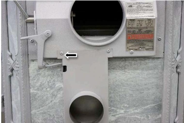
6. Secure the duct from the outside air source to the adapter. A hose clamp or sheet metal screws could be used depending on the type of duct.
