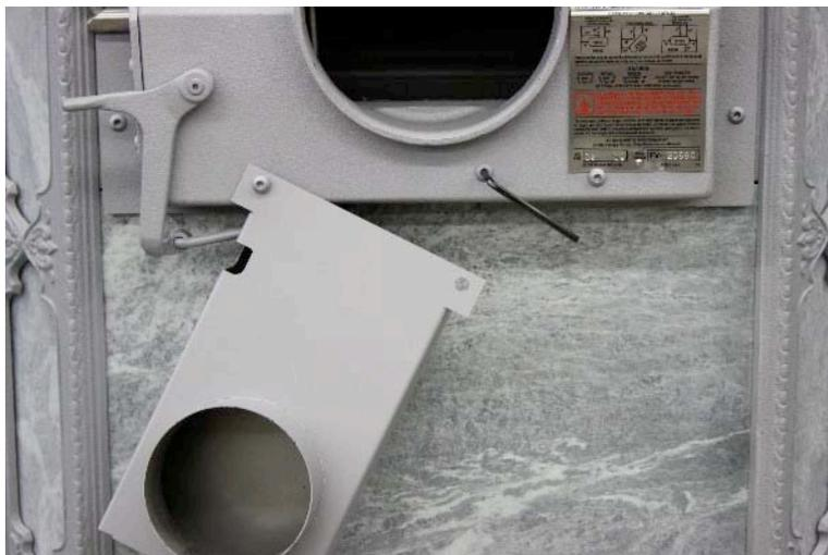
5. Secure the adapter to the flue collar with the button head bolts previously removed. The shorter bolt should be closest to the damper handle.
