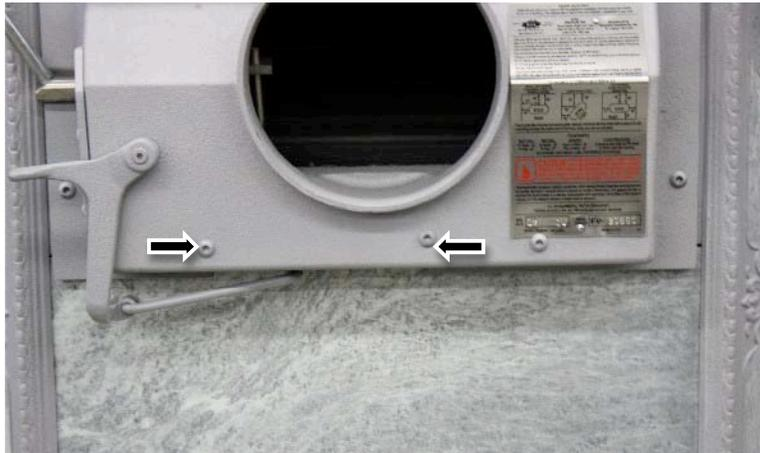
3. Use a 5/32" allen wrench to remove the bolts.
