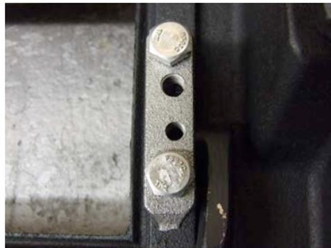
22. Once the retainers are fastened securely start the "adjustment" screws in the center of each retainer, but only by a thread or two. Now lift the bypass cover from the bottom side upward so that the two pivot points or "bull horns" are pressed up against the bottom side of the retainers. With the cover held in this position, tighten the
