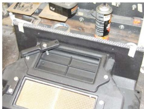
29. Let the gasket sit for about three minutes to allow the glue to become tacky enough to hold gasket in place when the combustor pan gets turned right side up.
