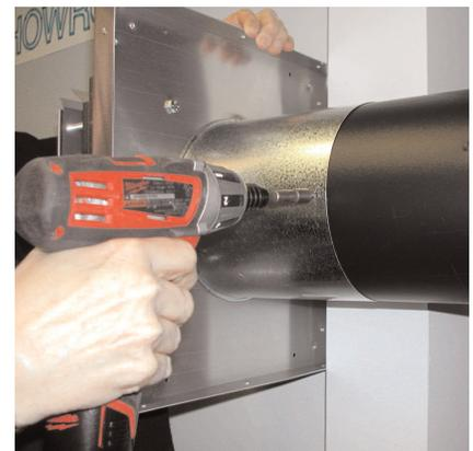
Last piece of pipe is pushed into vent cap and screwed in place - **not** twist-locked
