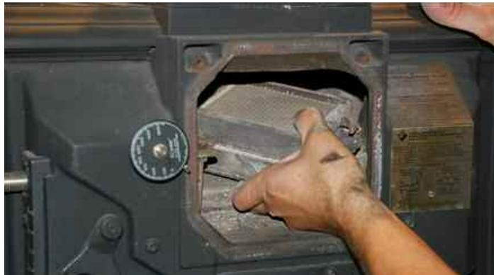
Replacing the combustor in a Keystone stove. The combustor can be removed through either the back flue collar or the cover plate.
