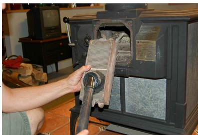
means removing it from the stove and cleaning off ash deposits with a soft brush or shop vac. When you're done, just put it back into the stove.
