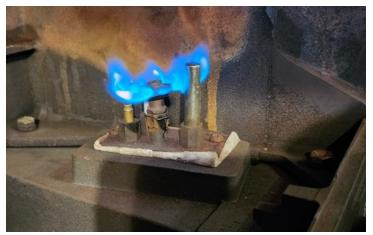
The pilot orifice is located under the round cap. The pilot orifice has two holes in the bottom to let air in, and a small gas outlet at the top, under the round cap.
