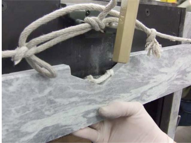
9. To replace the under the front stone simply lift it to remove and then place the new one in position.
